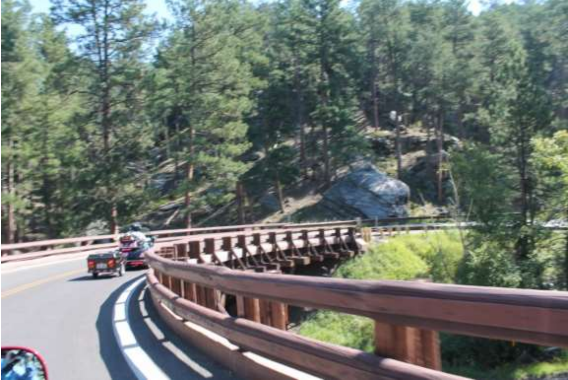
Iron Mountain Road
